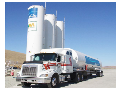
LCNG fueling stations
