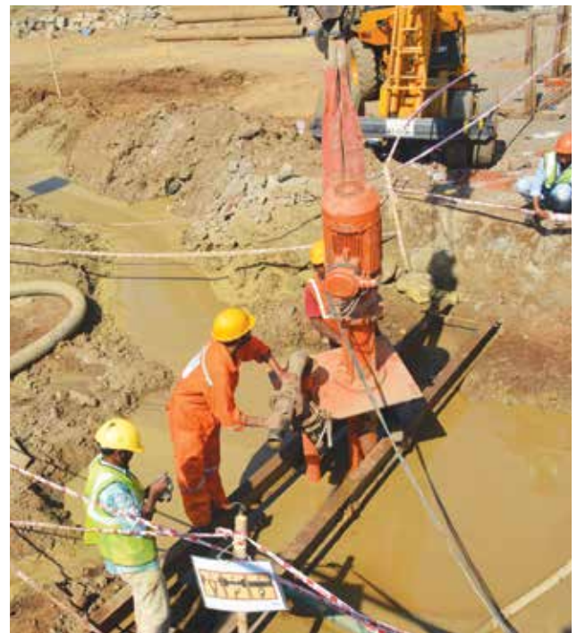
MGL work site.
