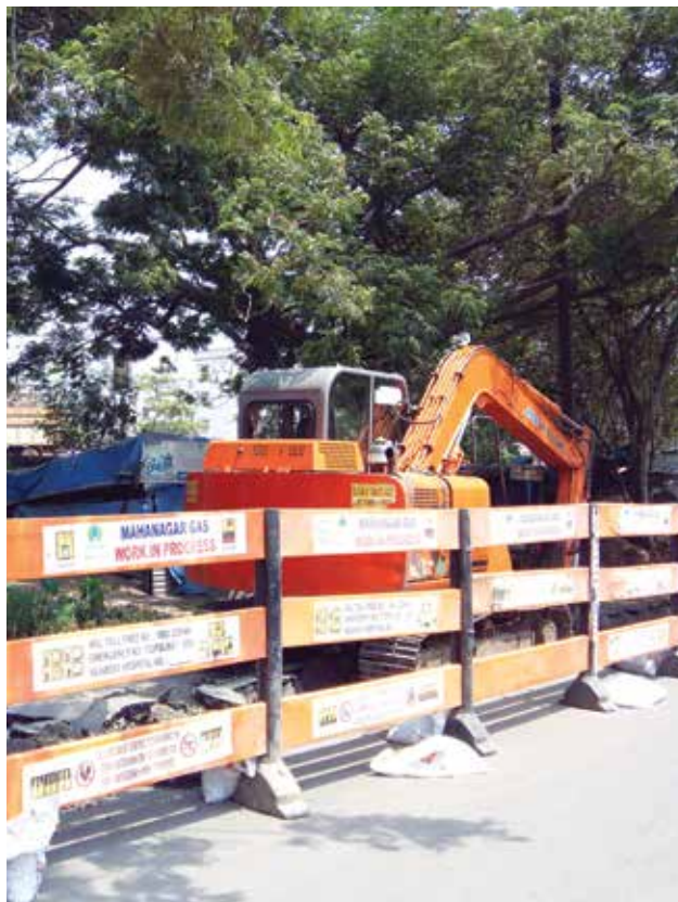
MGL work site
