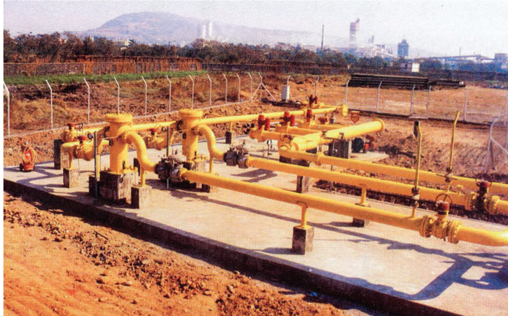
Construction of City Gate Station at Wadala
