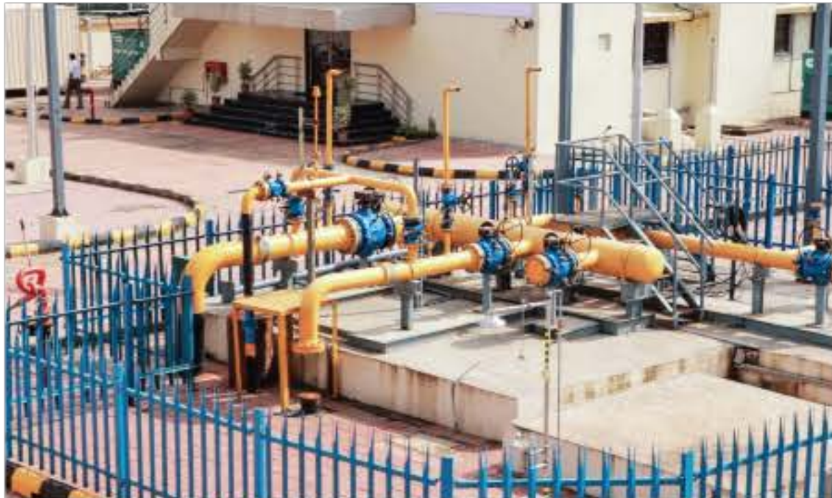
City Gate Station, Taloja
