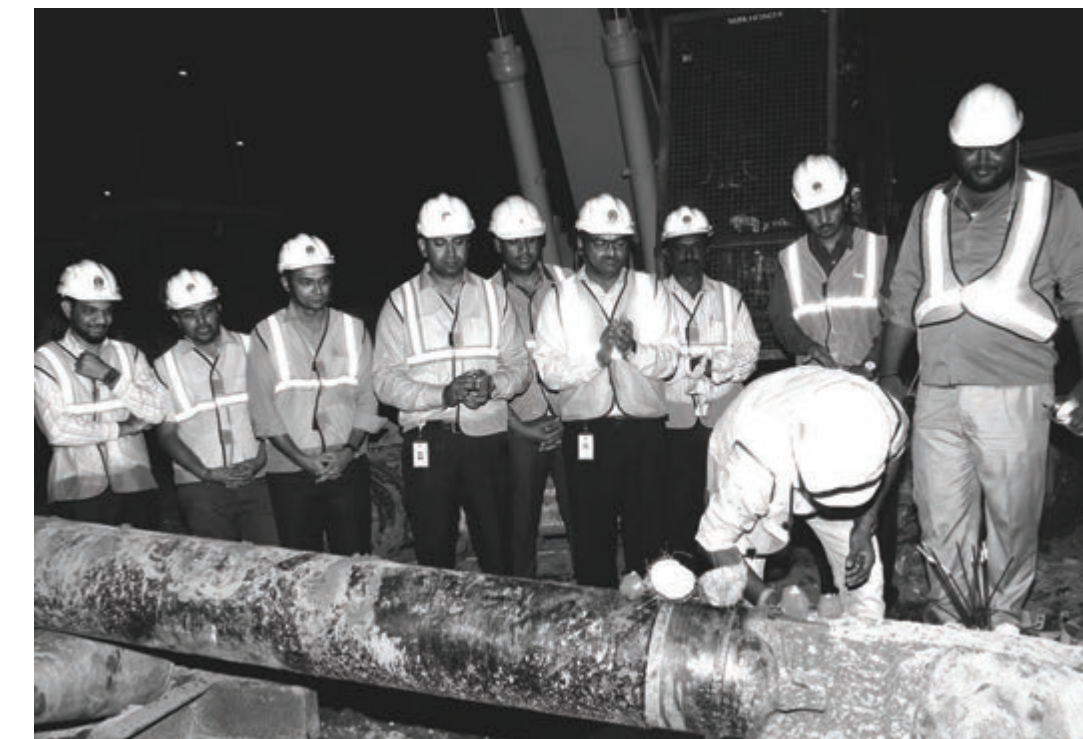
Inauguration of Laying of Steel Pipeline by MGL team
